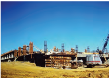
Founders Hall under construction
